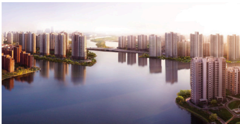
R&F PROPERTIES, TIANJIN, CHINA
