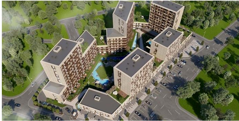
SUR YAPI TOPKAPI PROJECT, TURKEY
